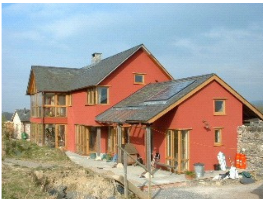
Figure 1: Taiffordd Fawr. This eco-house used professional builders, but the client managed the financial part of the project and was instrumental in the design and decisions to include eco-features, such as solar water heating, PV panels and wood pellet boiler. Architect, Pat Borer
