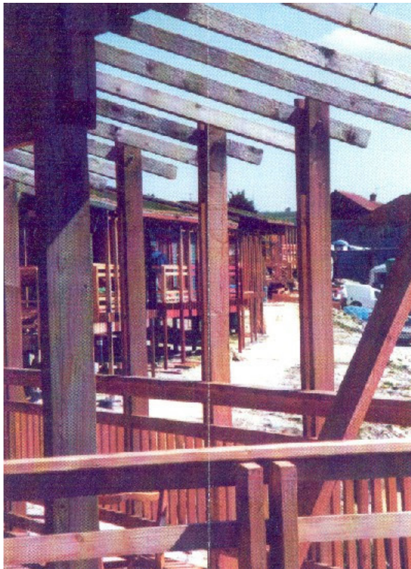
Figure 3: Hedgehog Self-Build project in Brighton, consisting of ten detached bungalows
