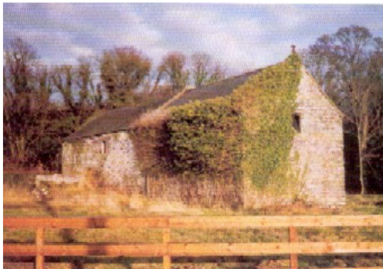
Figure 4: Before and after pictures of eco-barn conversion, N. Ireland
