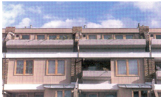
Figure 3: Angell Estate after renovation works
