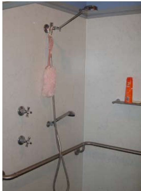
3. Completed shower rebuild. Where appropriate, advice is sought from local Occupational Therapists to ensure modifications suit the tenants' needs.
