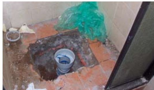
2. Leaking showers are stripped, water-proofed and rebuilt.
