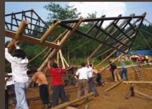
Post-Earthquake Reconstruction and Rehabilitation in Da Ping Village China
