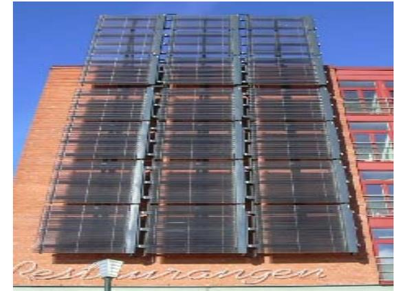
*Building-integrated solar thermal system*
