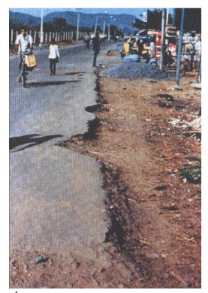
Conventional building methods of raising roads result in rapidly eroding edges as heavy rainfall washes away the sub-base. 50 per cent of all conventional road building goes to raising the roads and maintaining them.
