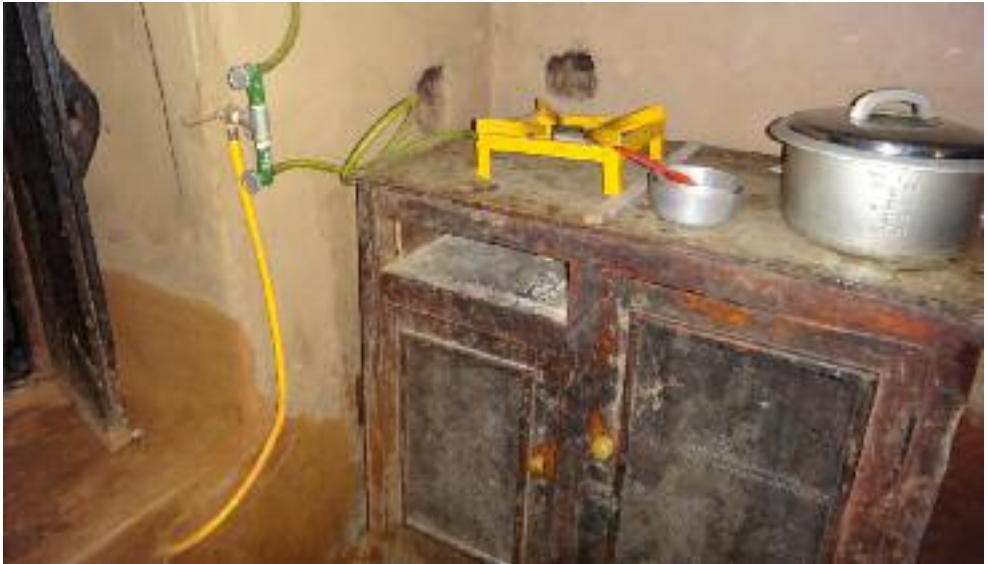
Cooking stove and pipes connected to the biogas system
