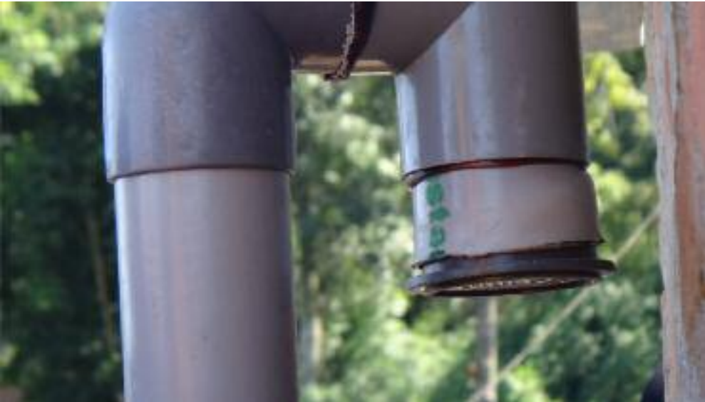
Pipe attached to the roof collecting water run-off for storage
