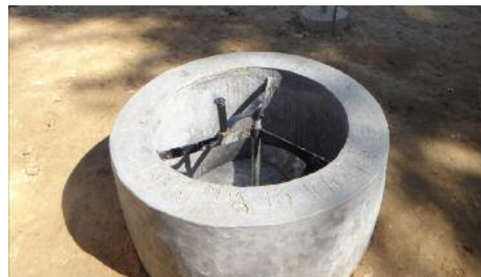
A newly built biogas digester
