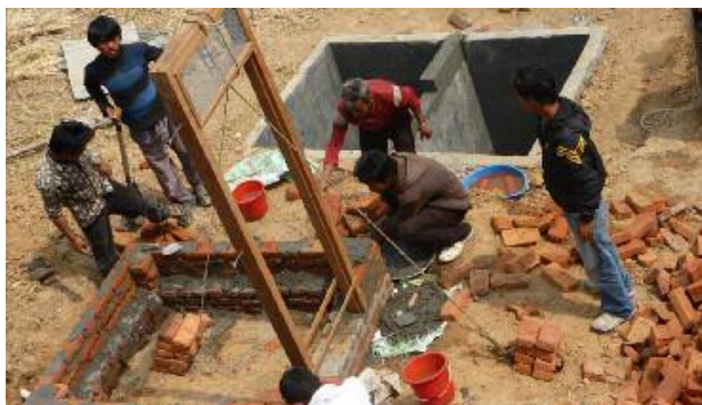
Toilet and waste system construction in Nepal
