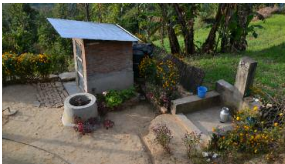
An integrated waste system: toilet, rainwater storage, septic tank, biogas digester
