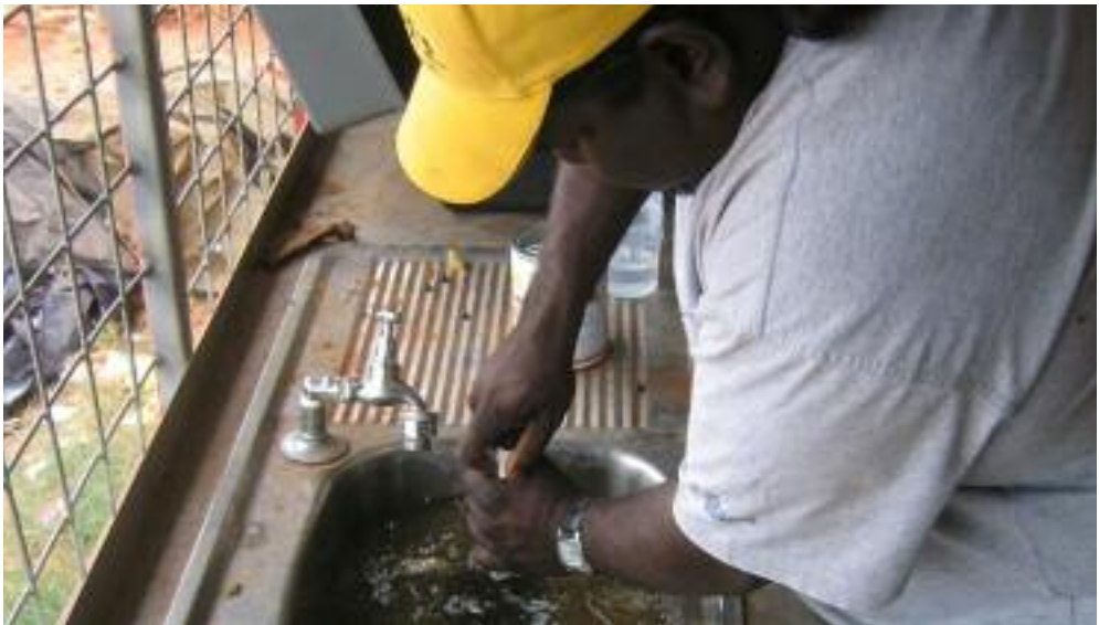
Fixing a wastewater blockage
