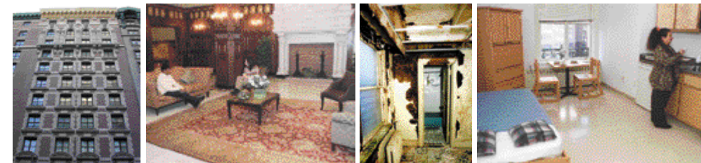
Common Ground Community – The Prince George Before After
